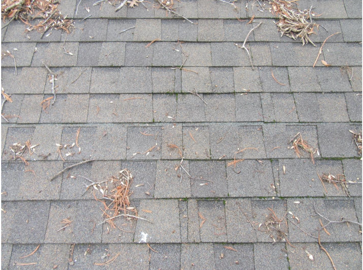
#24 Partial back side view where the shingles are marginally installed.
