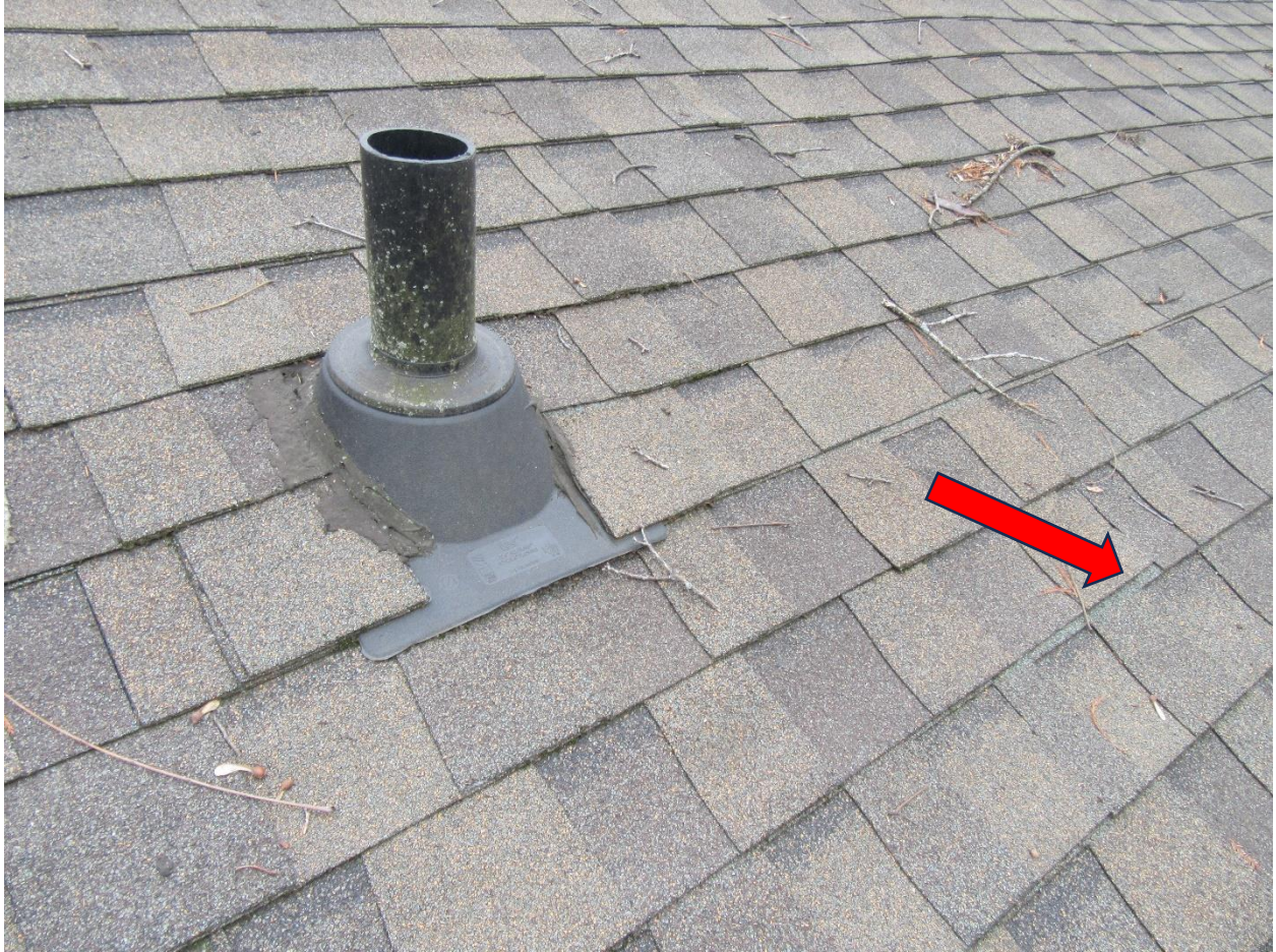
#17 Marginal quality shingle installation on part of the back side. Some rows are uneven.
