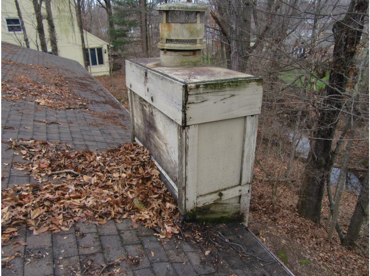
#18 Chimney view. The leaves prevented a proper inspection. Chimney wood siding is in very poor condition and will require replacement.
