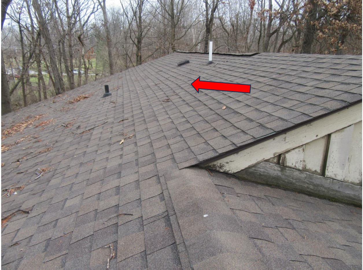
#26 Partial back side view reveals the slightly crooked shingle rows and the slightly uneven roof structure.
