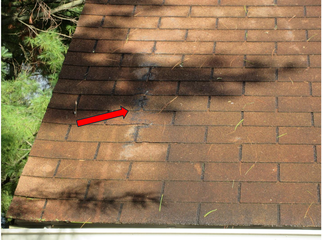
#16 Shingle damage on the N/W corner roof area. Damaged shingles should be repaired or replaced.
