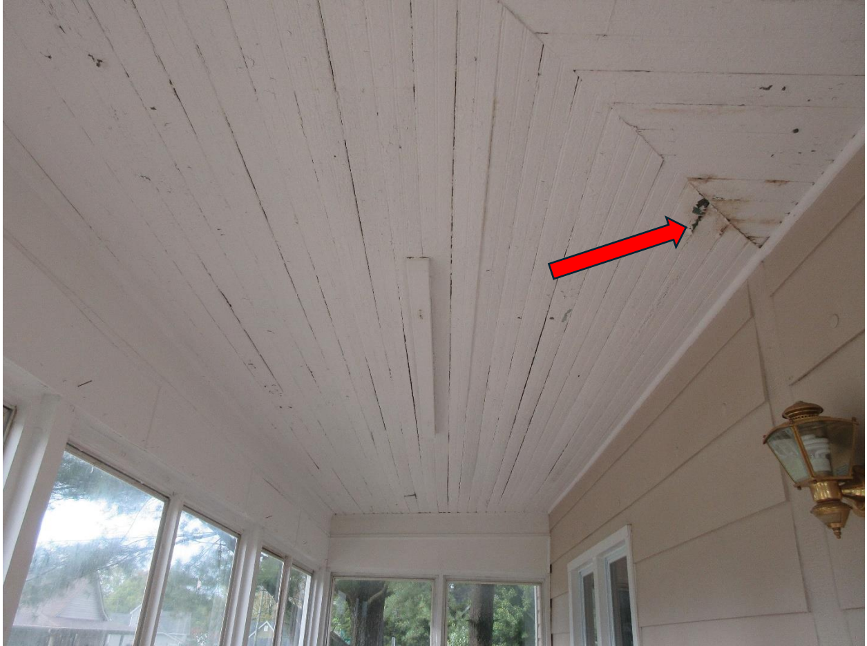
#32 View of the front porch ceiling. Water stains and damage appear to be a result of a metal roof leak issue above.
