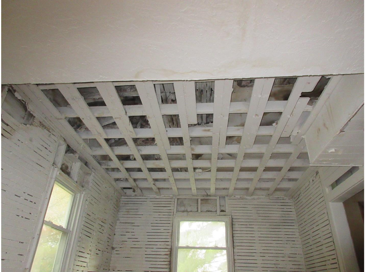
#39 Ceiling view in the east room that may have been the kitchen or dining area. There is significant roof structure and roof damage above. This is where it appears a tree fell on the house.
