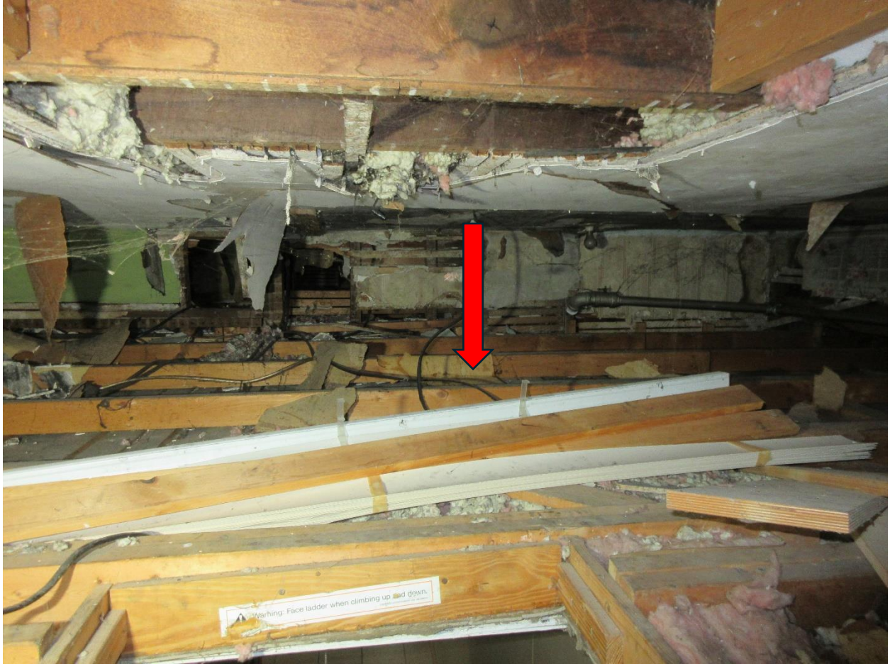
#42 The interior ceiling has been lowered about two feet from the original ceiling.
