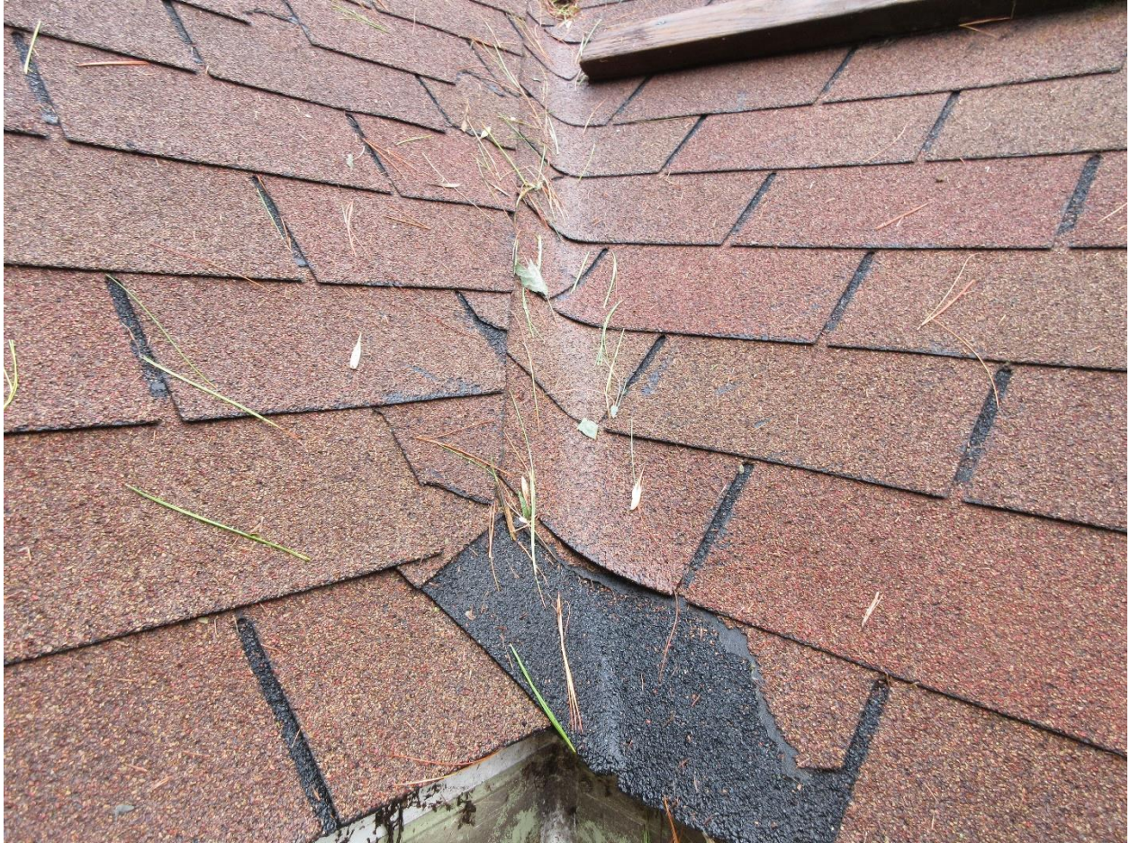
#30 Damaged shingles in the lower S/E corner roof area. Damaged shingles should be repaired or replaced.
