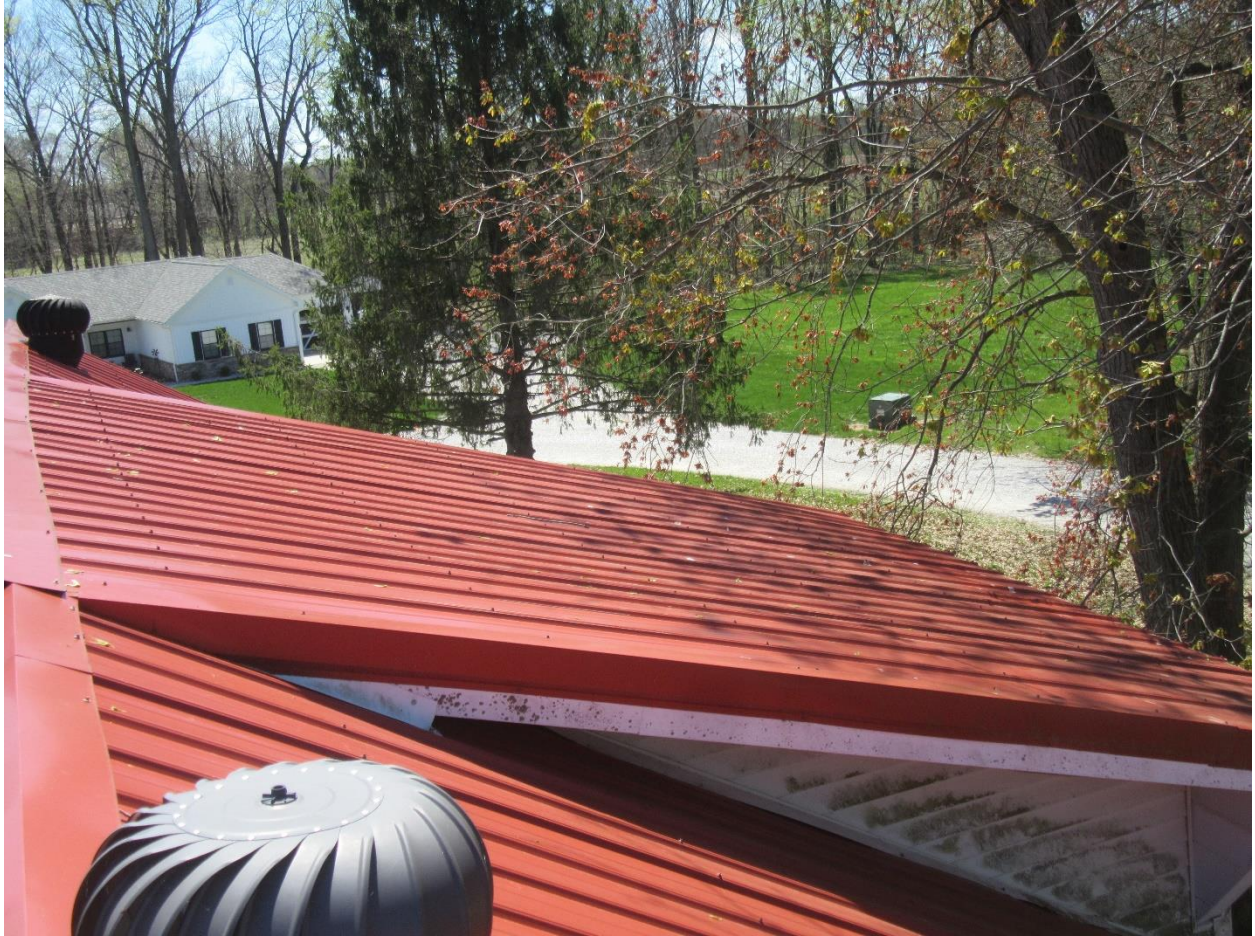
#11 View of the west side center roof area.
