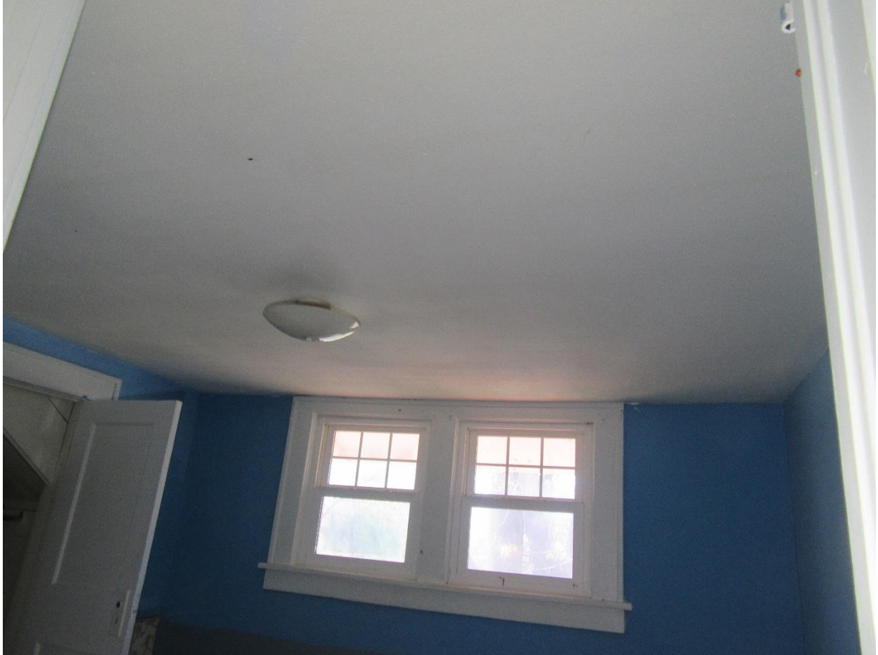
#27 Upper level west side room. I did not detect leak issues.
