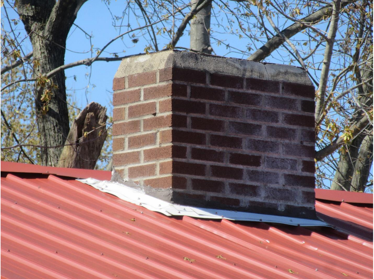
#23 Close-up view of the chimney.
