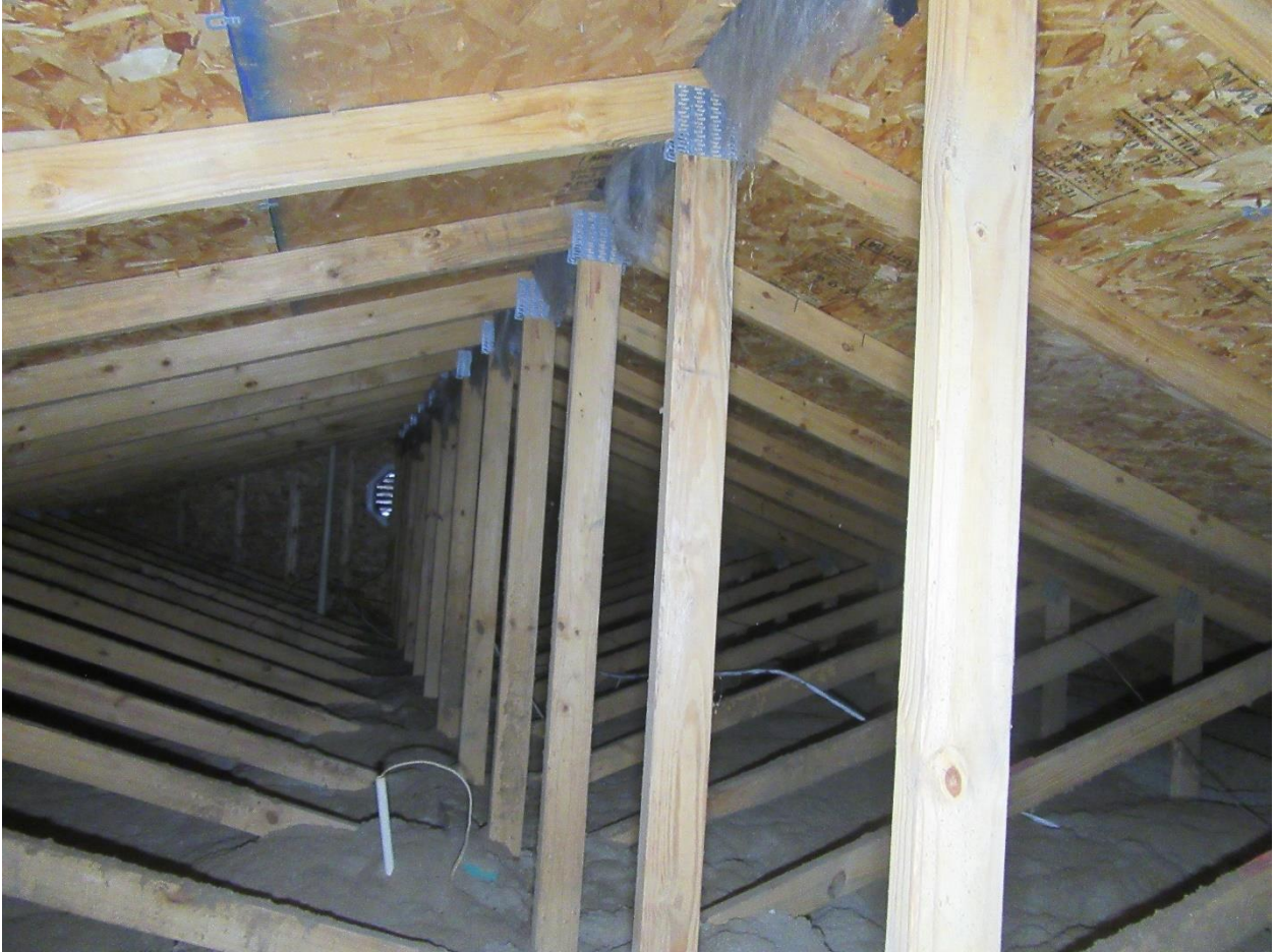
#43 Detached garage attic view. I did not detect roof leaks.
