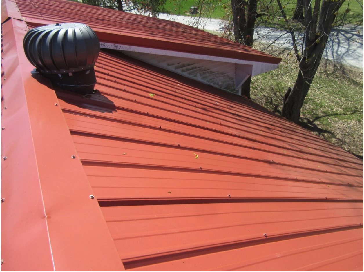
#10 Partial west side main roof view.
