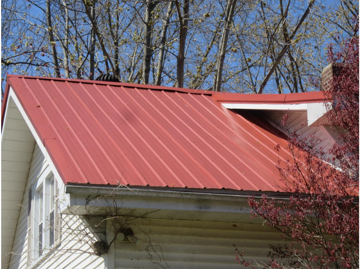
#17 View of the S/E corner of the roof.
