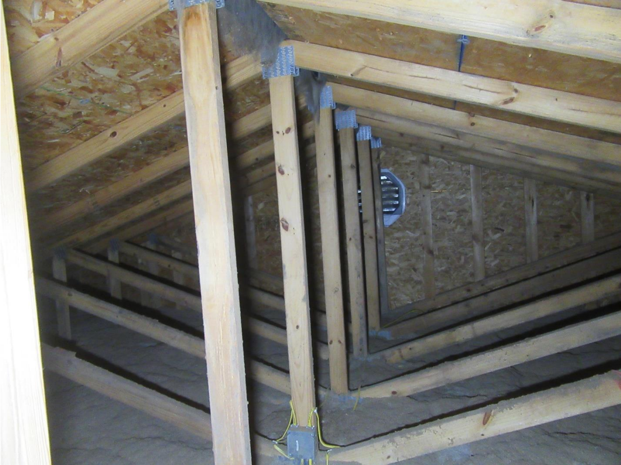
#44 Detached garage attic.
