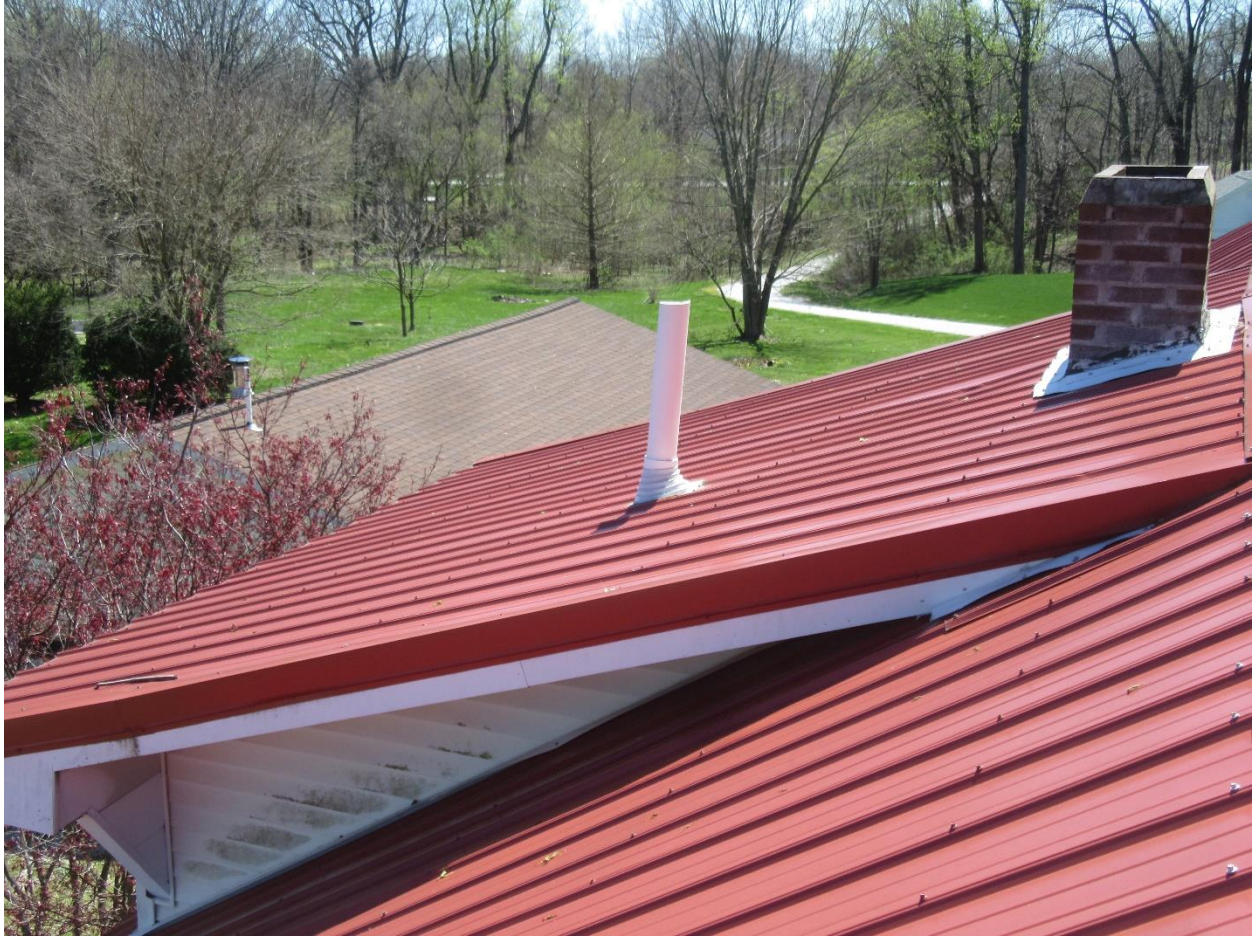
#12 View of the east side center roof area.
