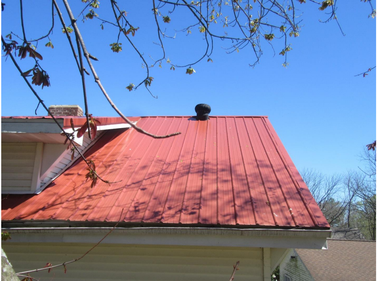
#18 View of the S/W corner of the roof.
