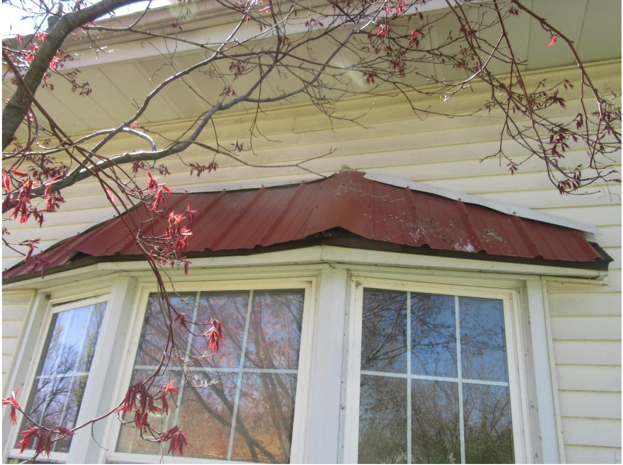
#21 View of the small east side roof area.
