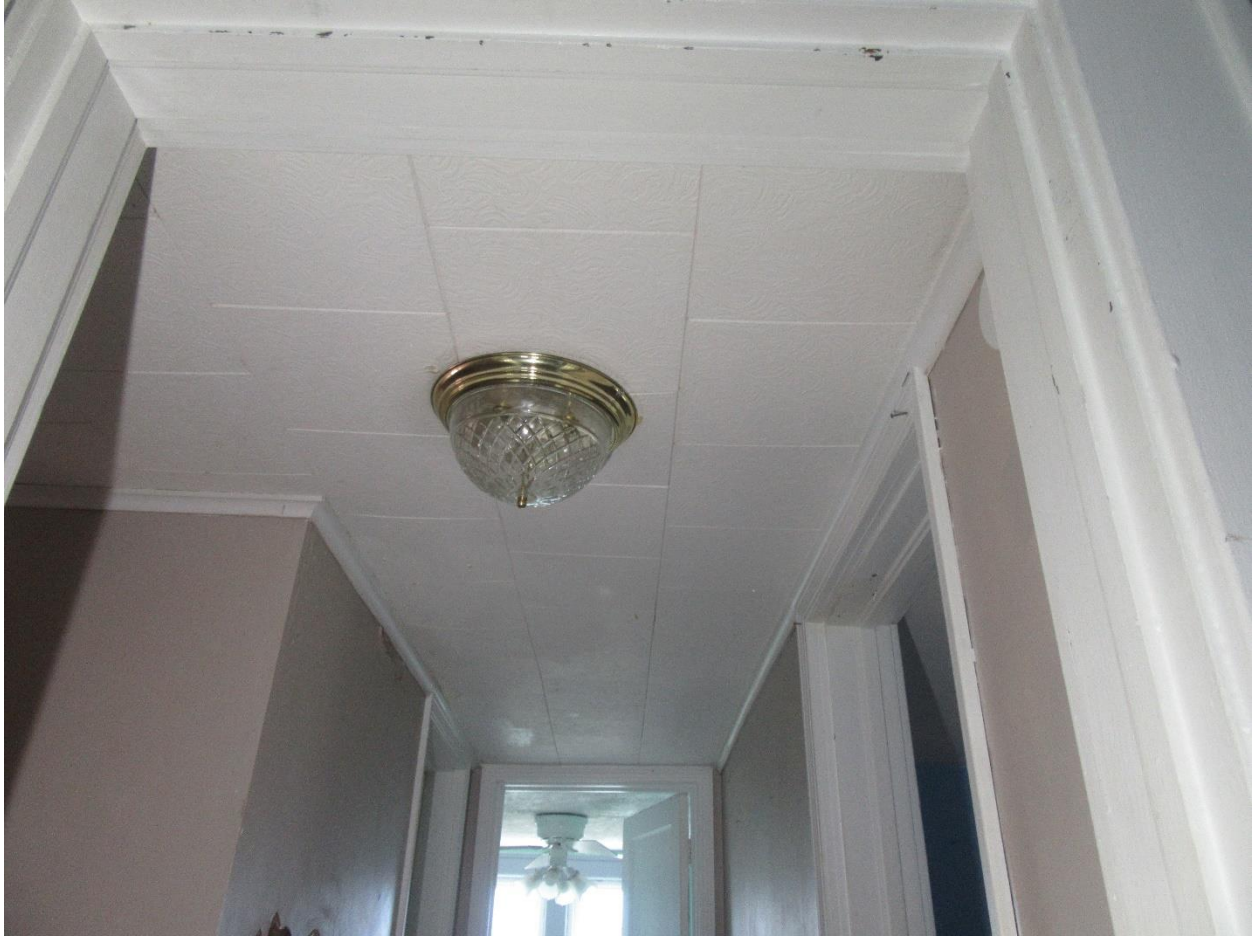
#26 Upper level hall view.
