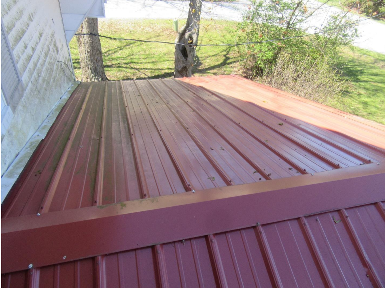
#5 Front porch roof view on the west side.
