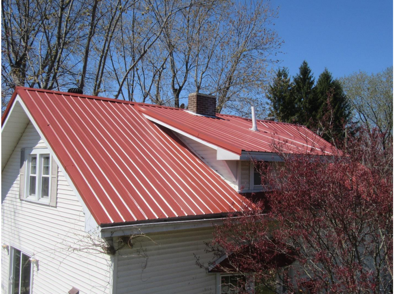
#22 East side roof viewed from the garage roof.
