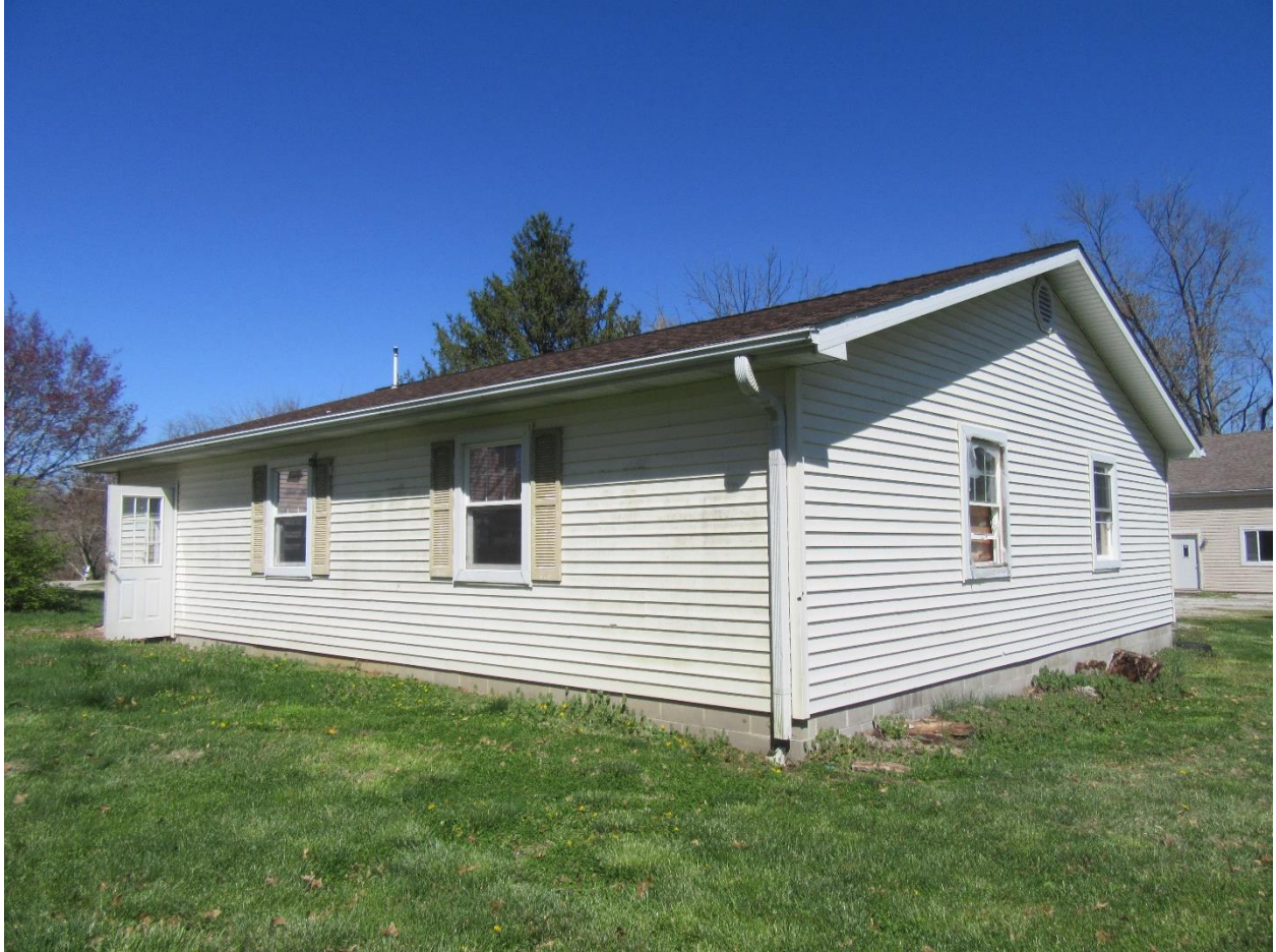
#35 Detached garage building.
