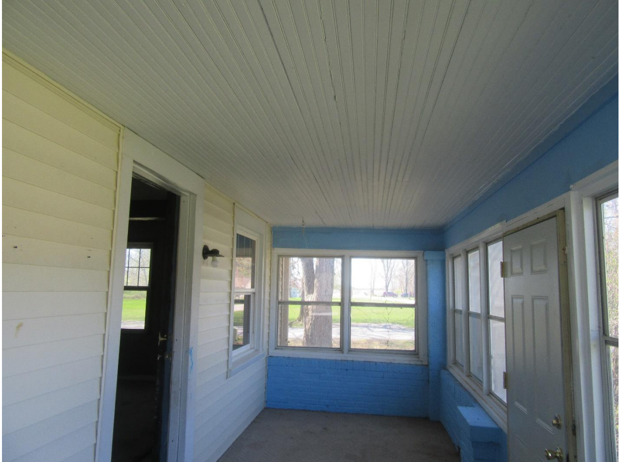
#24 Front porch view. I did not detect leak issues.
