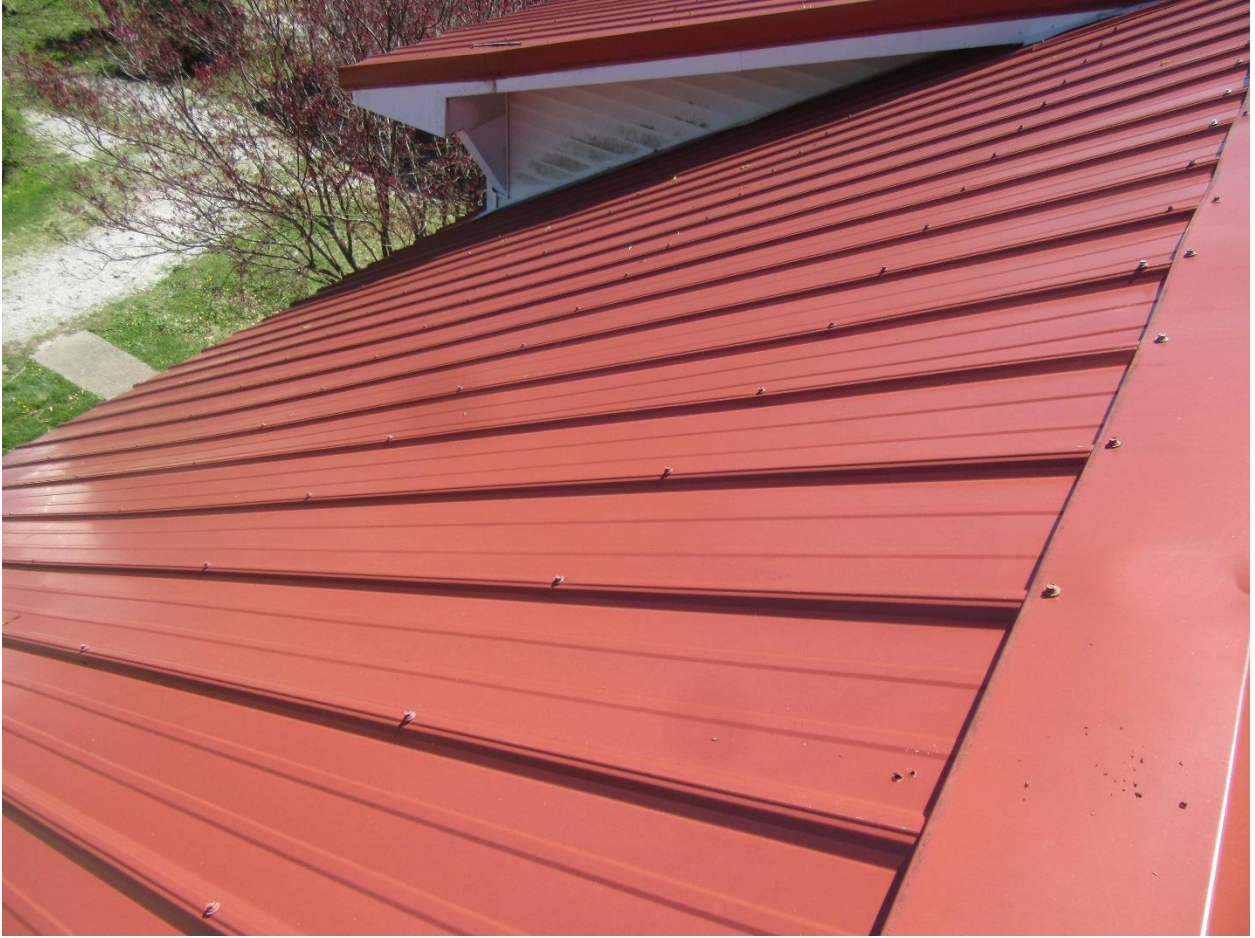
#9 Partial east side main roof view.
