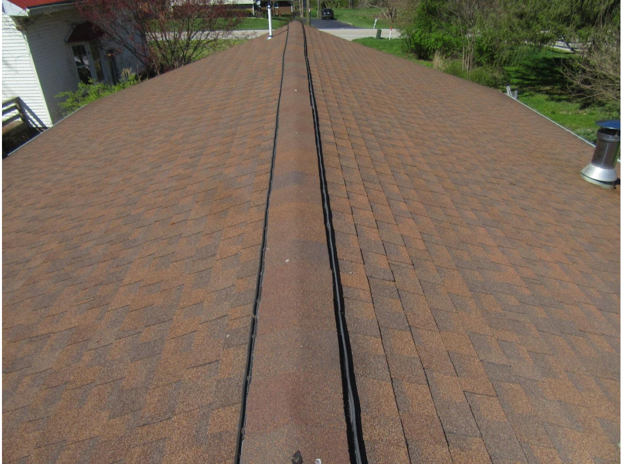
#37 Detached garage building roof view looking to the north end.
