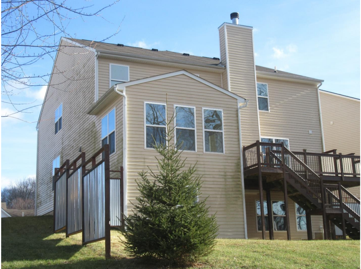
#5 Back side and partial south end view.
