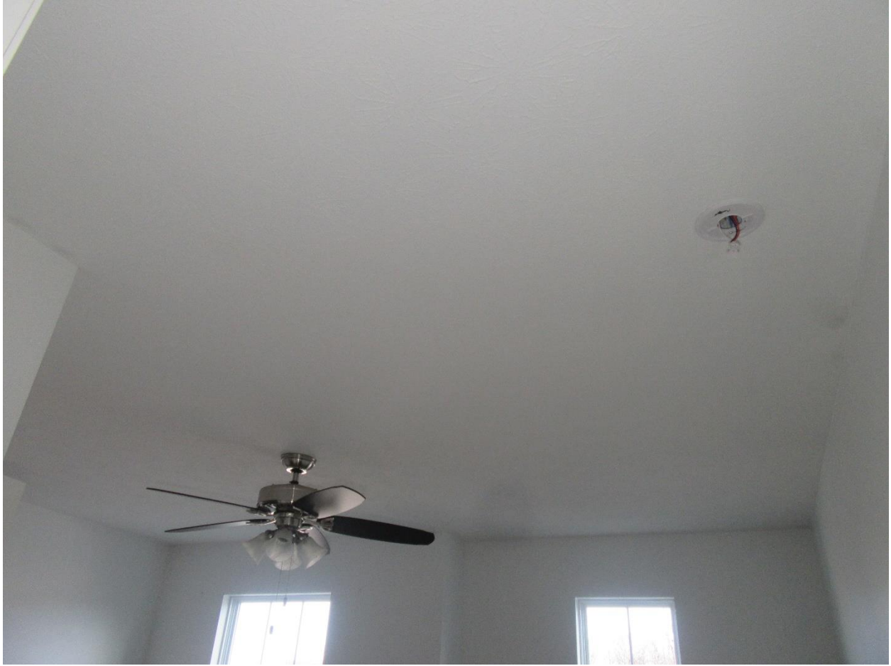
#30 Upper level front N/E corner bedroom ceiling view.
