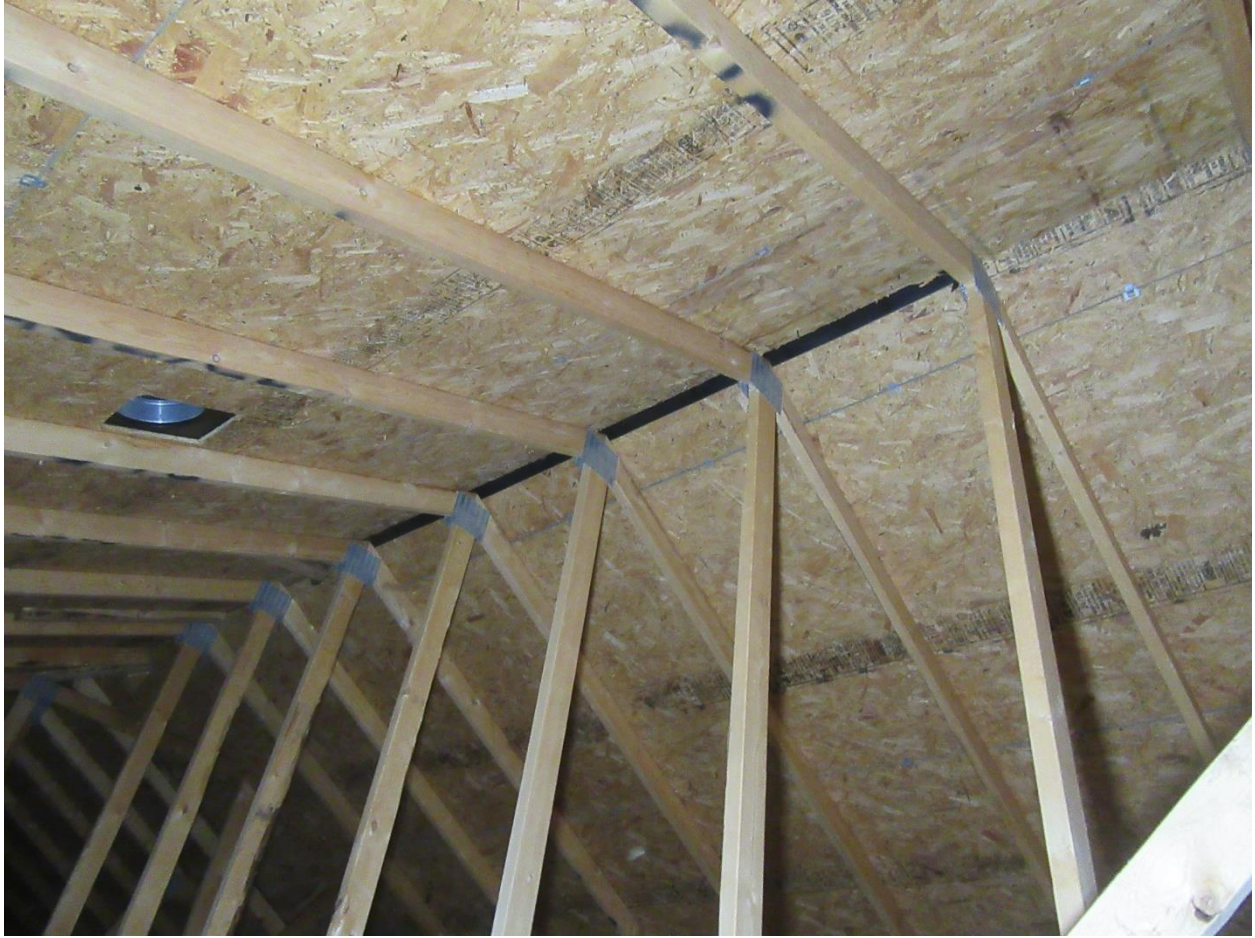
#46 Attic view in the center peak area.
