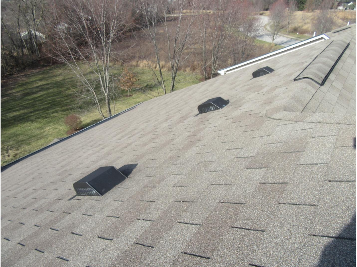
#11 Upper back side roof view of the N/W corner area.
