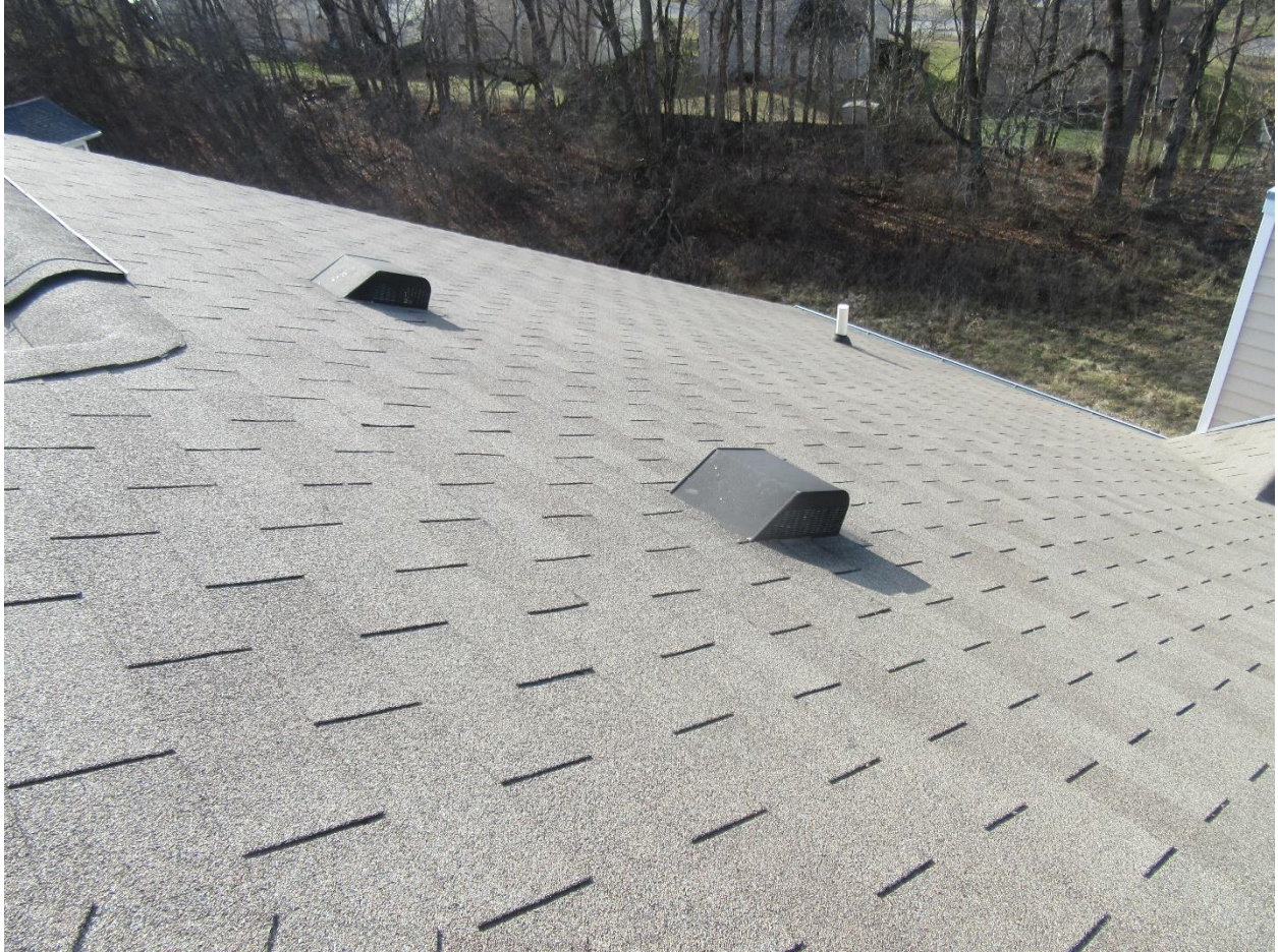
#13 Upper back side S/W corner roof area.
