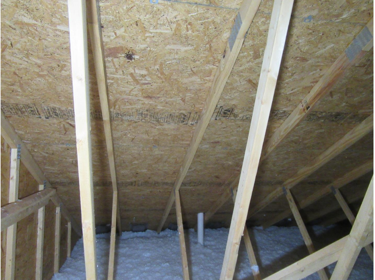
#45 View in the S/W corner attic area.
