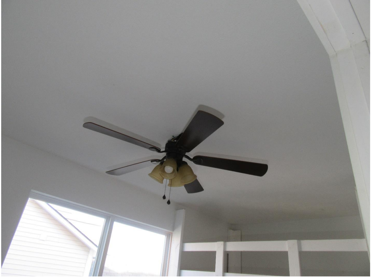
#31 Upper level south side center bedroom ceiling view.
