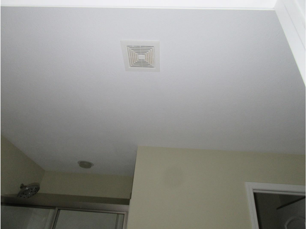
#37 Master bathroom ceiling view.
