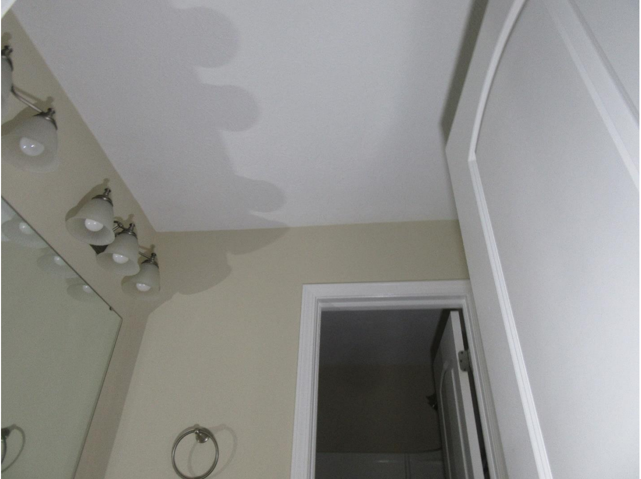
#36 Upper level center bathroom ceiling view.
