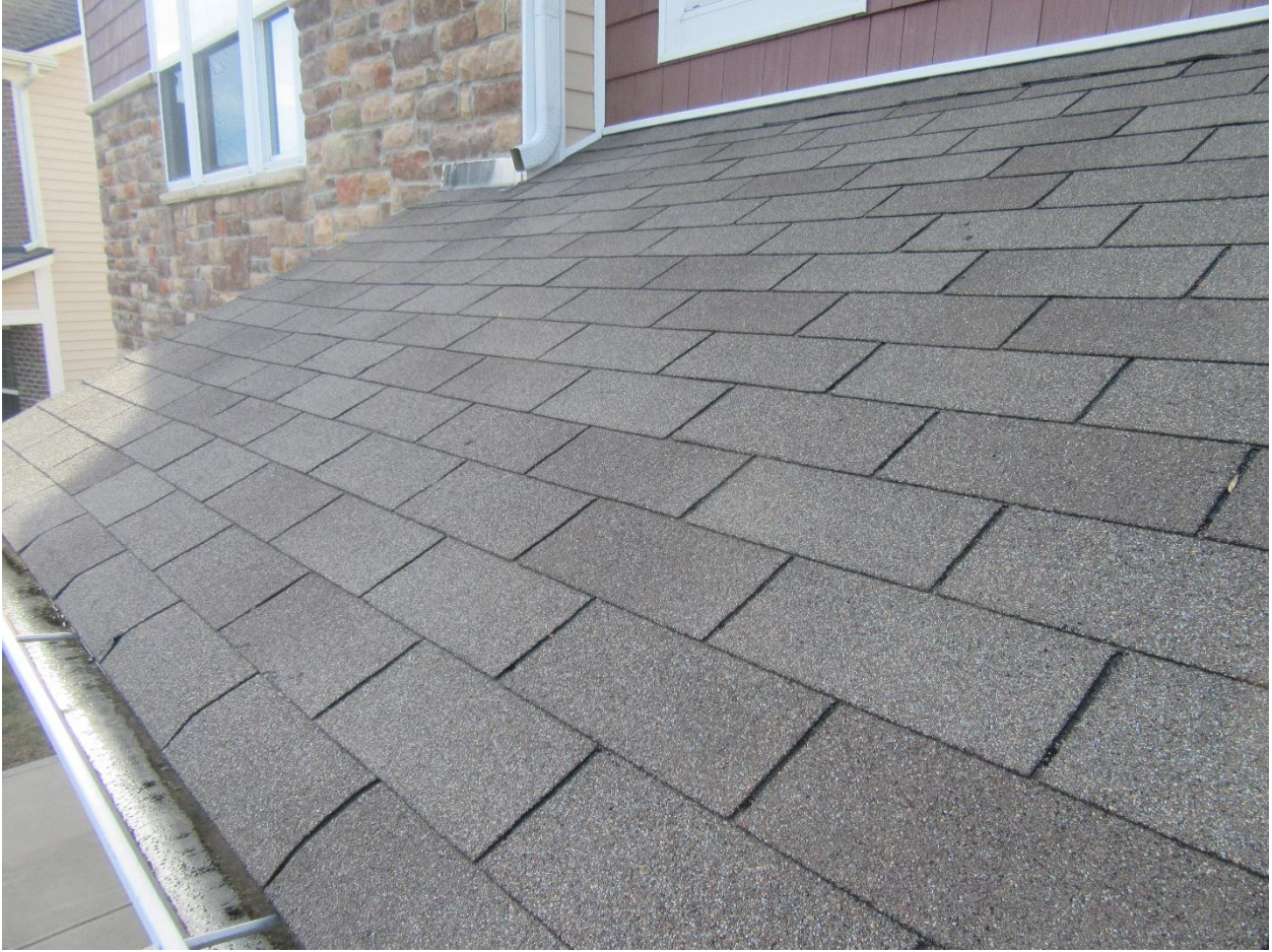
#24 Partial view of the front porch roof.
