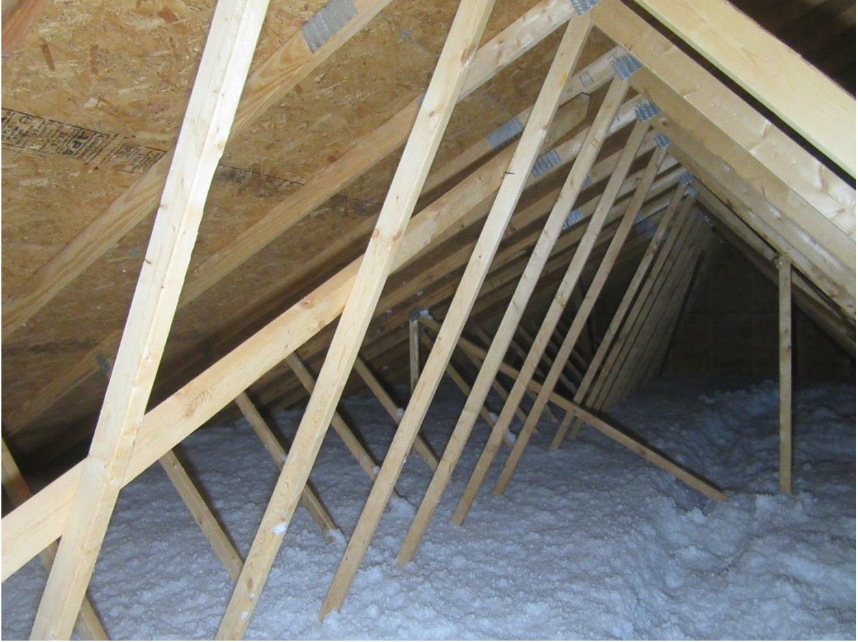
#44 View along the back side attic area.
