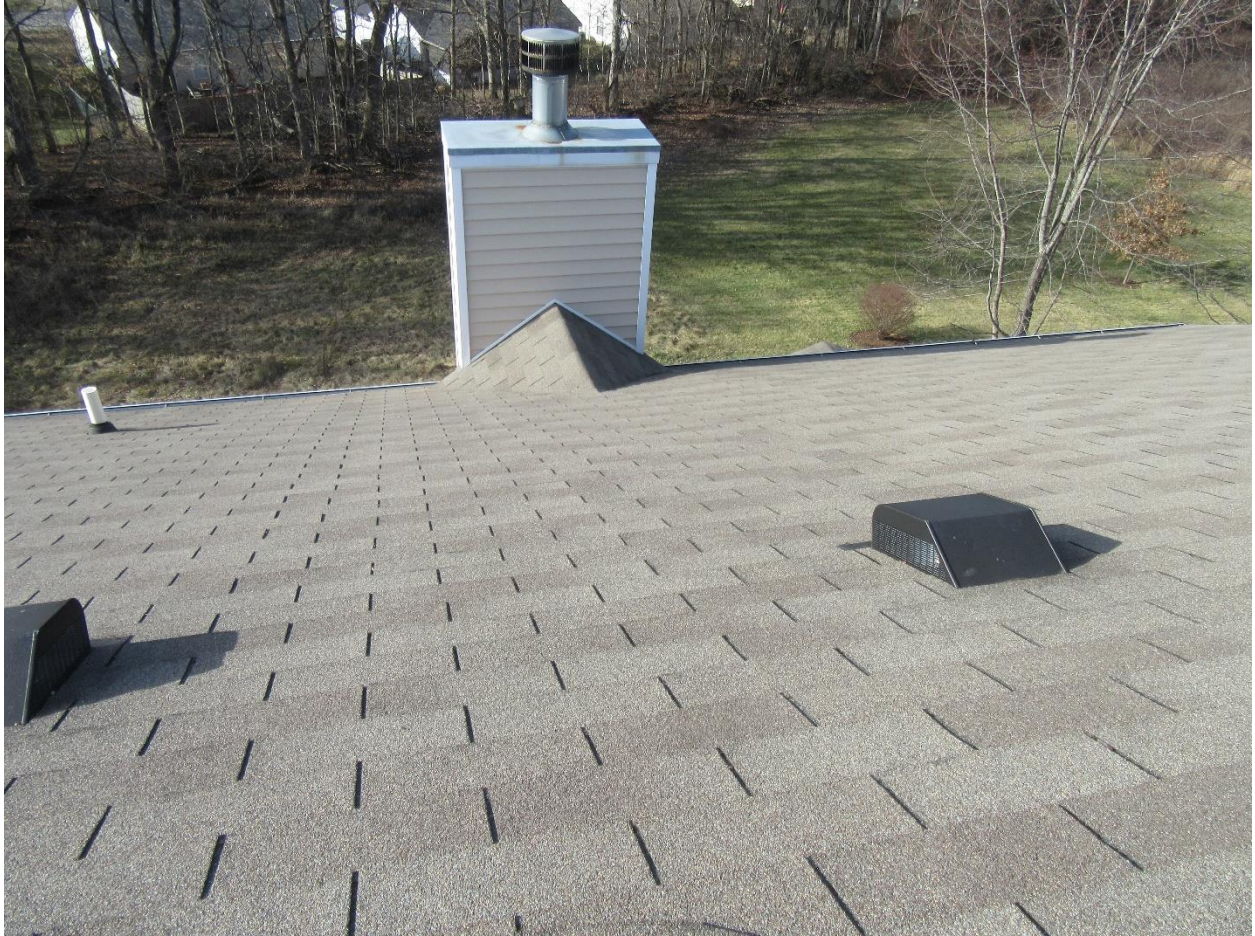
#12 Upper back side center roof area.
