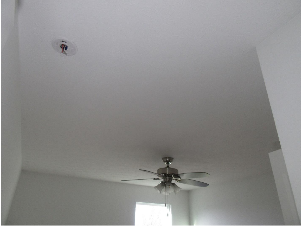
#32 Upper level N/W corner bedroom ceiling view.
