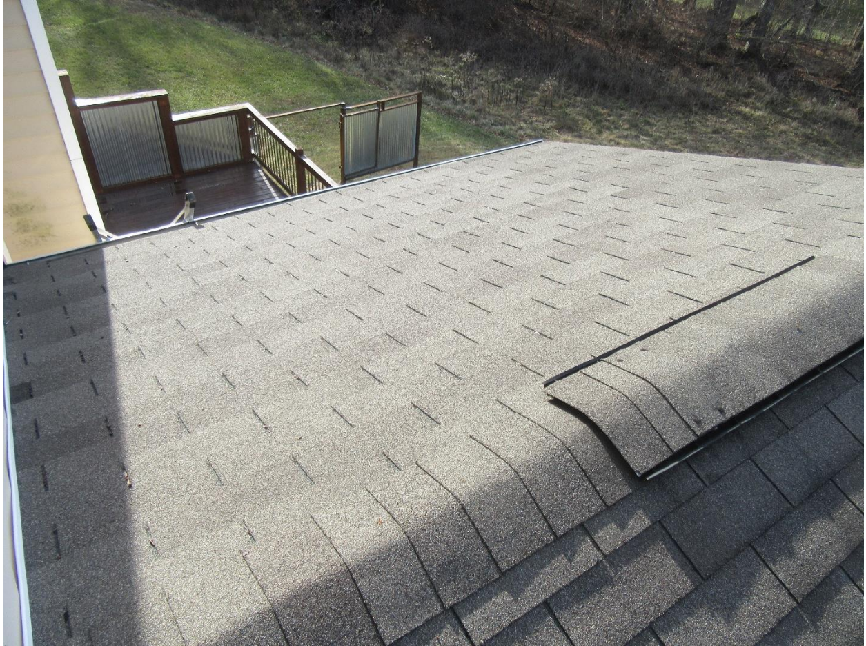
#21 Back side lower roof view.
