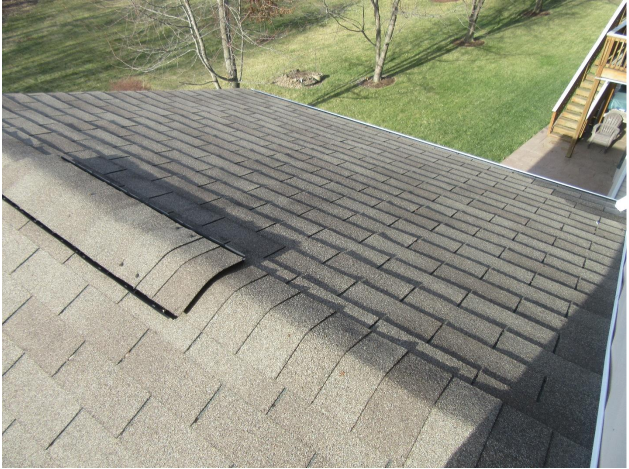
#20 Back side lower roof view.
