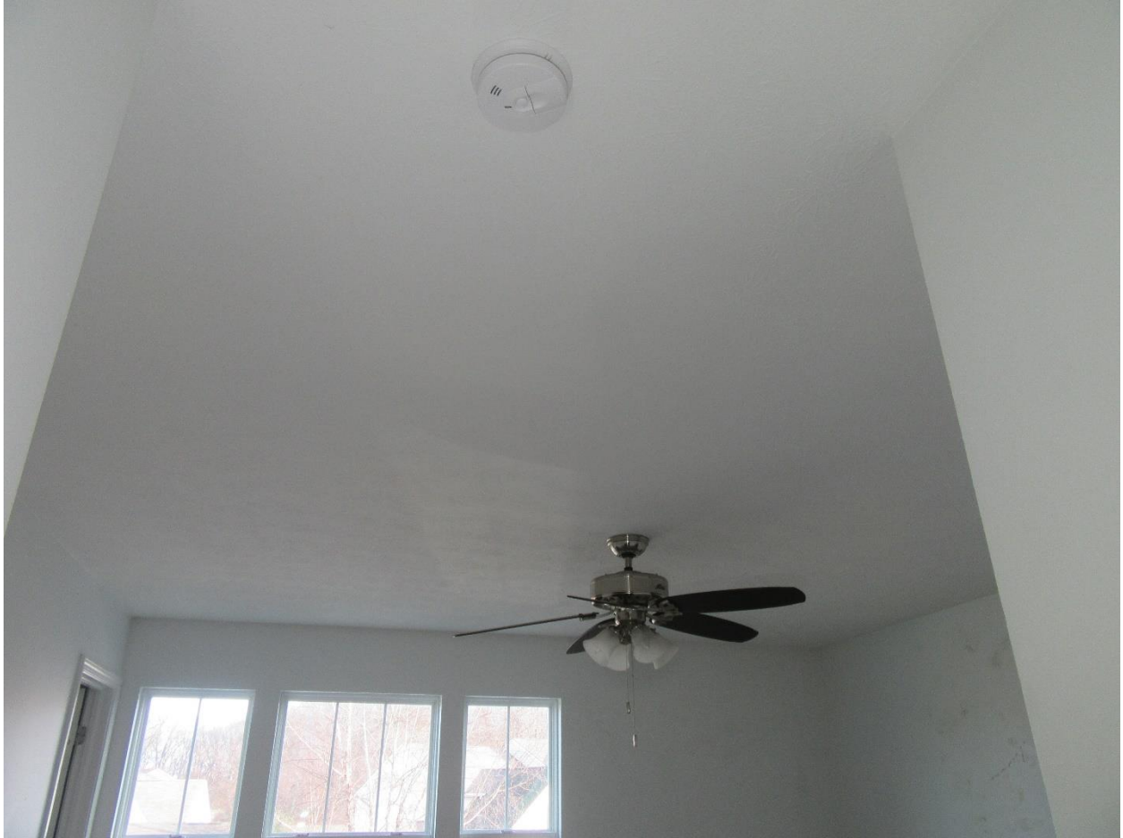
#34 Upper level front corner S/E corner bedroom ceiling view.
