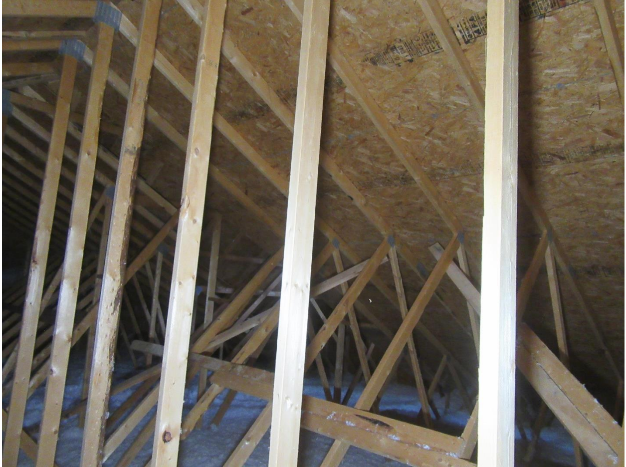
#43 View along the front side attic area.
