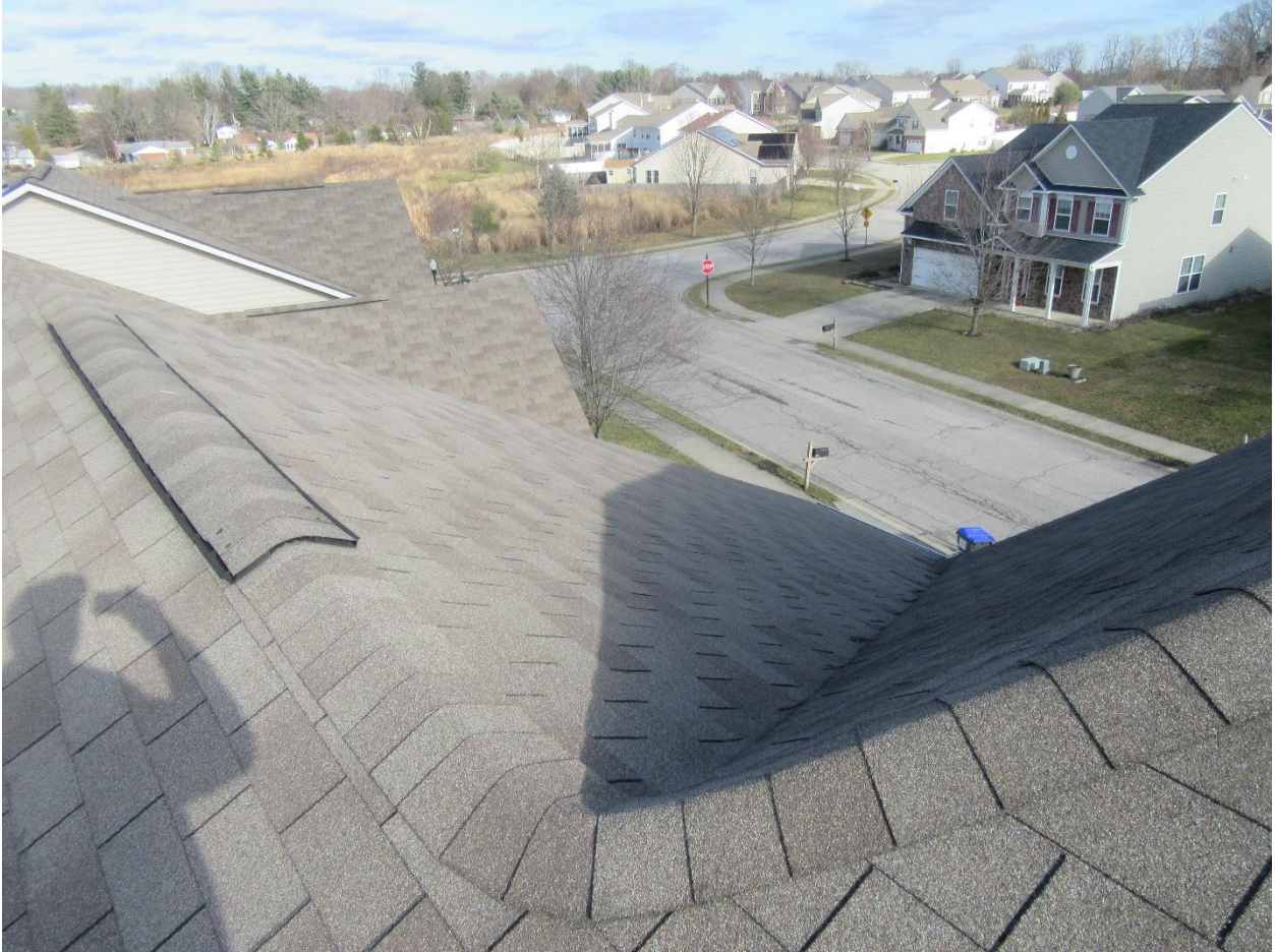
#7 View of the upper N/E corner roof area.
