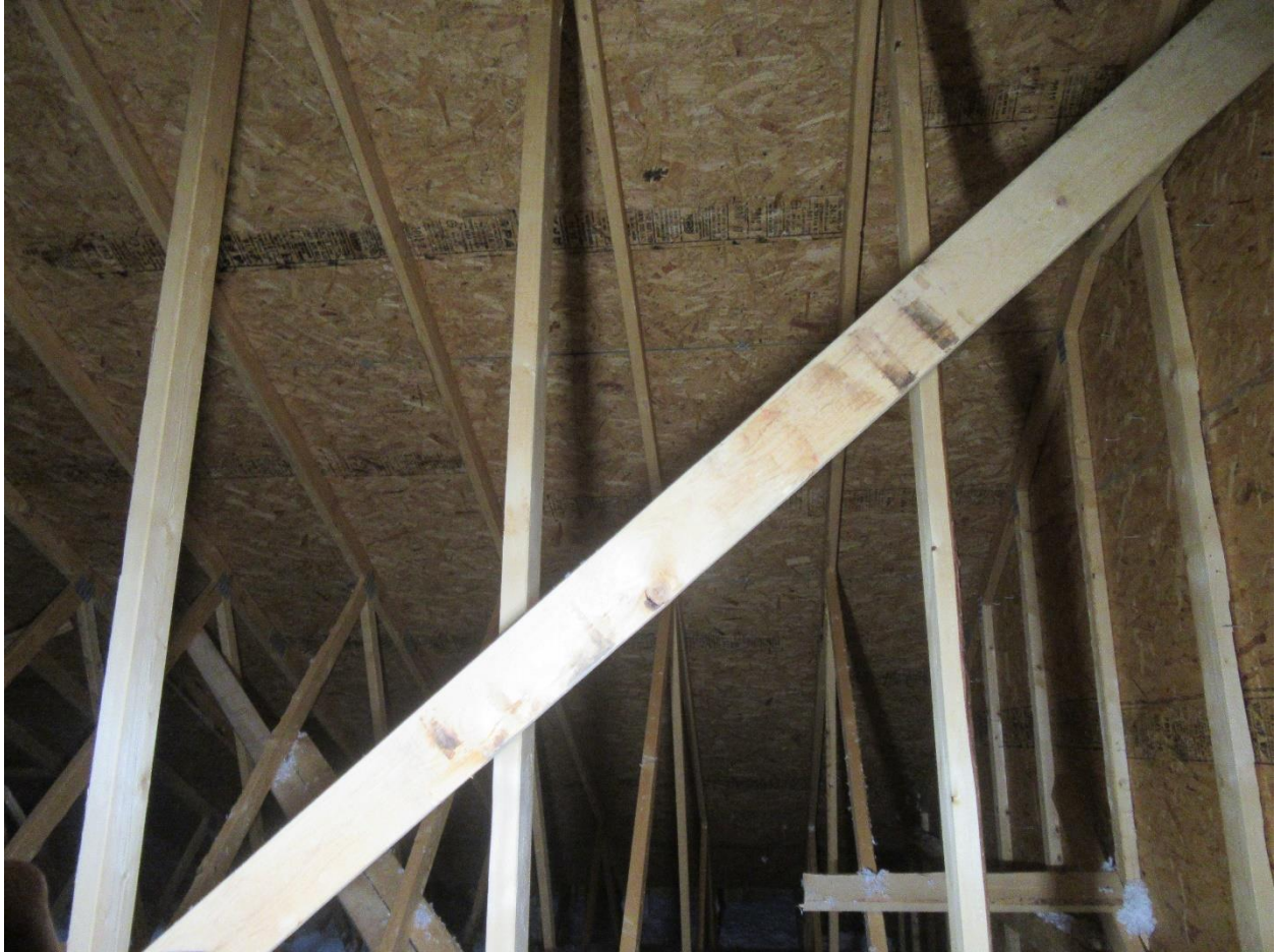
#42 View in the front S/E corner attic area.
