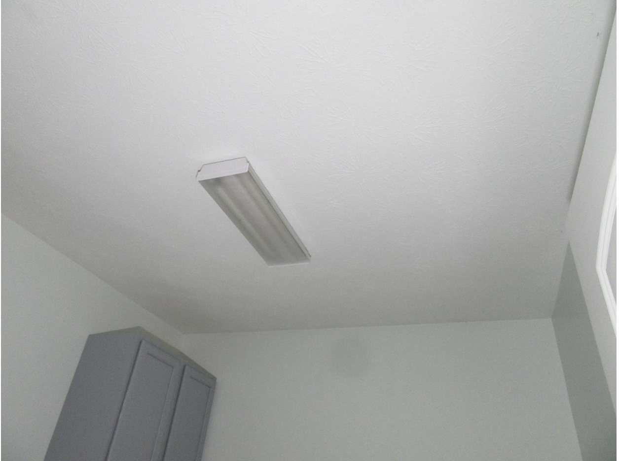
#35 Upper level laundry room ceiling view.
