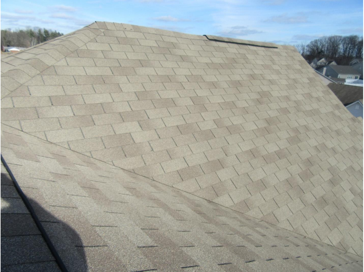
#10 View of the upper front center steep roof area.
