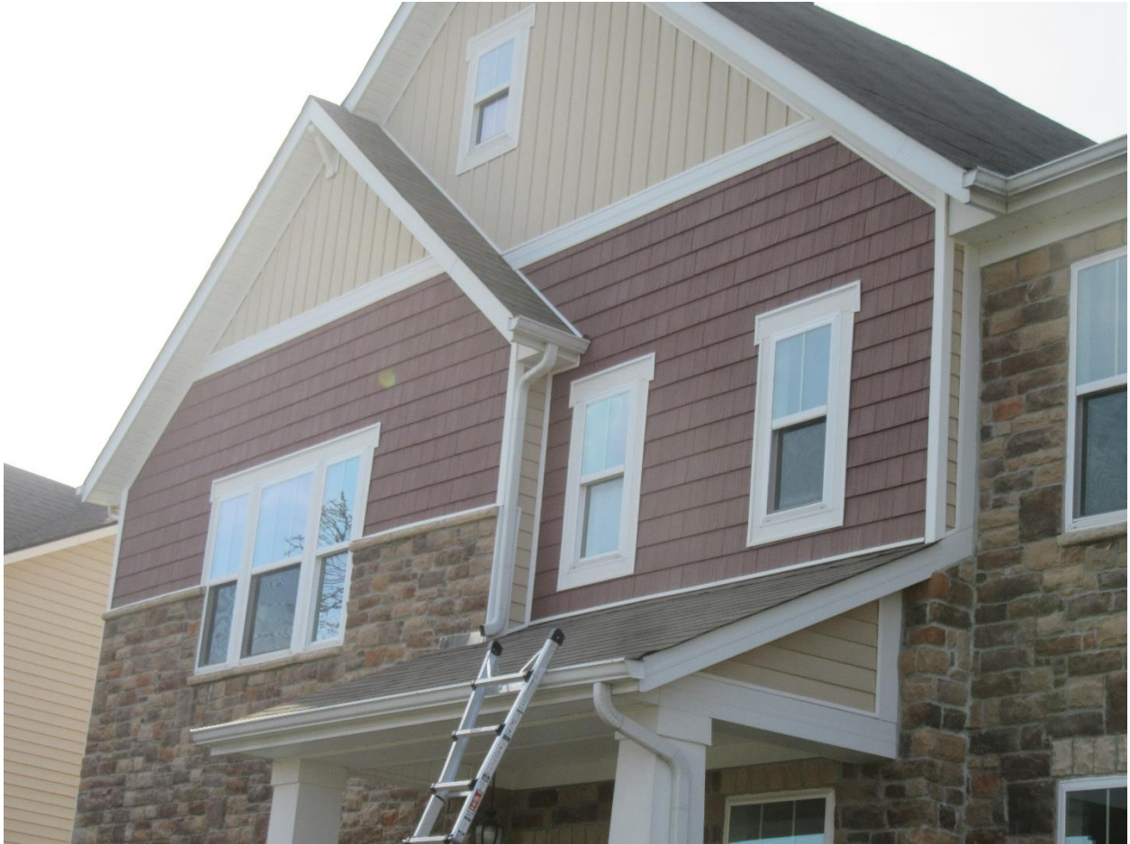
#26 View of the front porch and small front roof sections.
