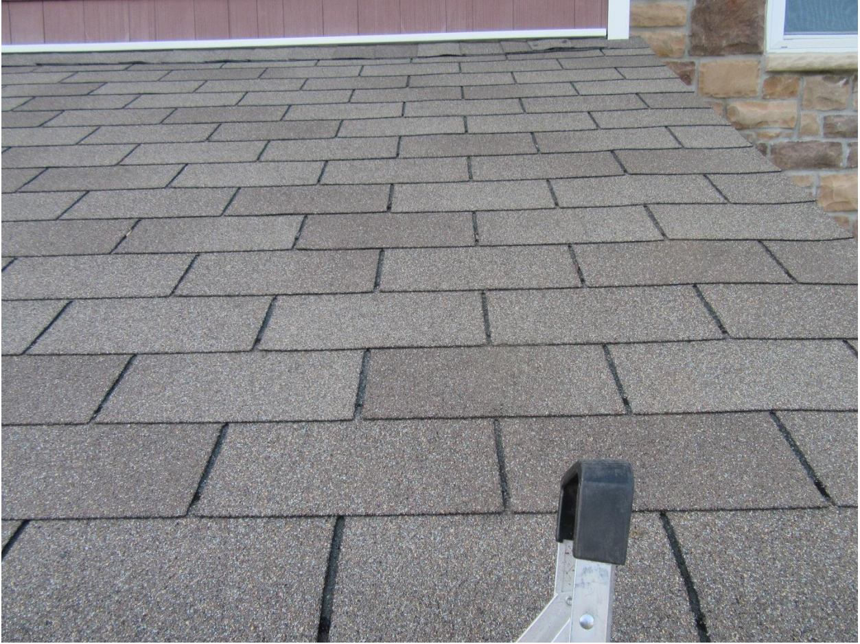
#25 Partial front porch roof view.
