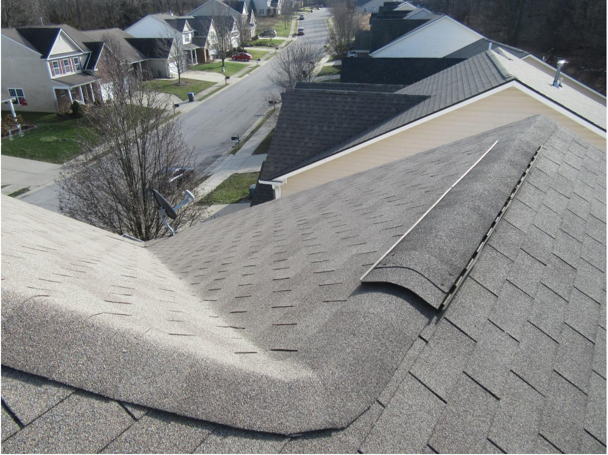
#8 View of upper S/E corner roof area.
