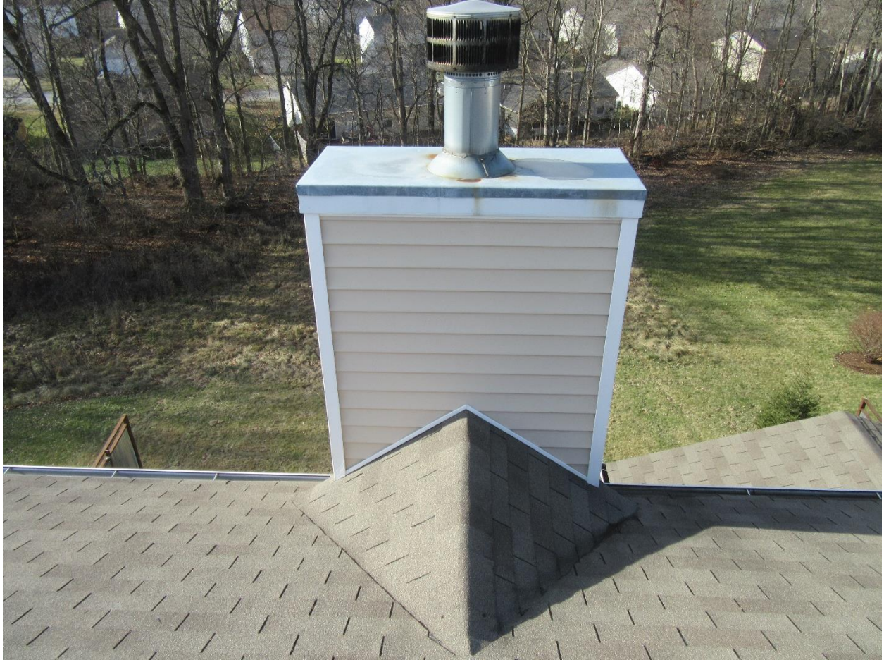
#14 View of the chimney and surrounding roof area.
