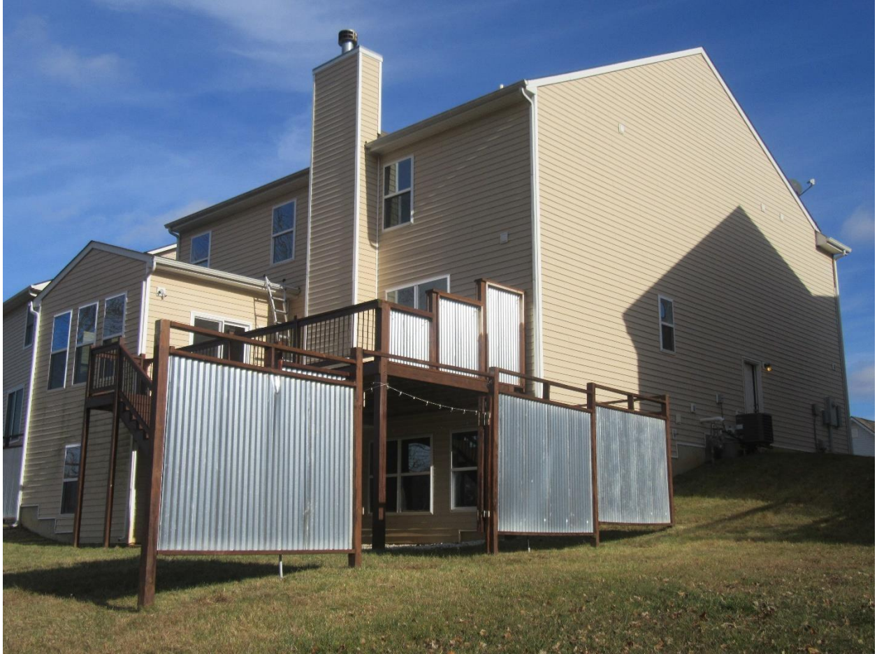
#6 Back side and north end view.
